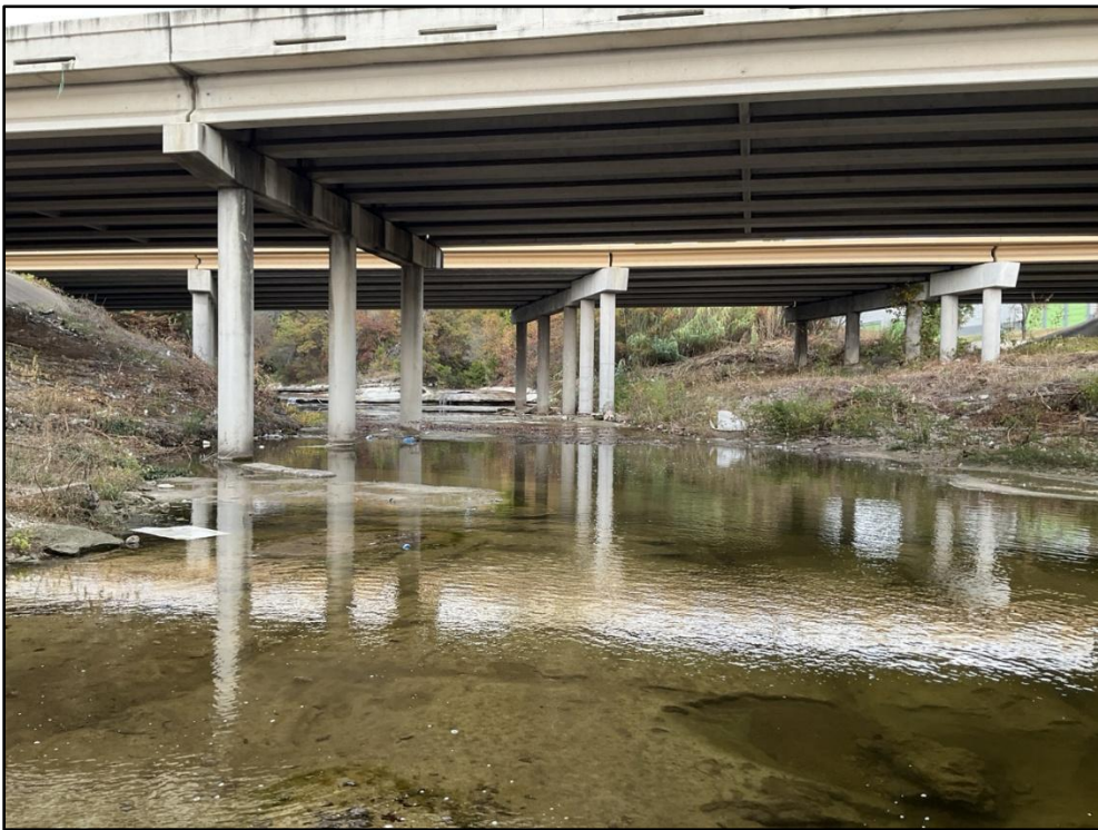
Photo 68 – STA 12+50 – Looking upstream at conditions under Highway 67; significant bedrock influence.
