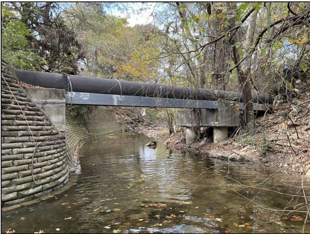
Photo 38 – STA 43+00 – Looking upstream at a 36-inch aerial sanitary sewer crossing. The crossing appears to be in good condition.
