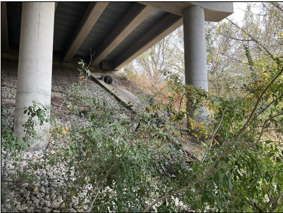
Photo 96 – STA 67+50 – 30-inch concrete stormwater outfall with flume on the left bank.
