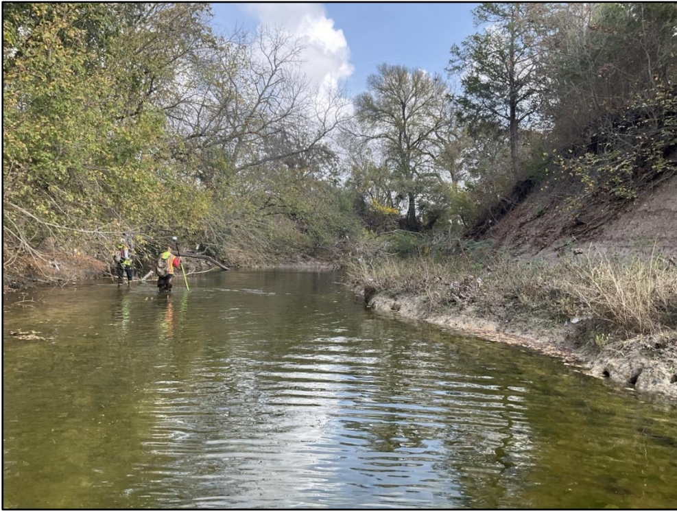
Photo 103 – STA 80+50 – Looking downstream, representative channel conditions.
