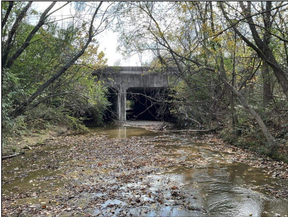
Photo 51 – STA 66+00 – Looking downstream at the East Danieldale Road culvert.
