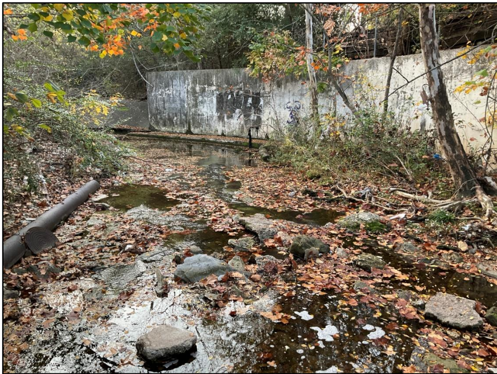
Photo 2 – STA 1+25 – Looking downstream from East Wheatland Road.
