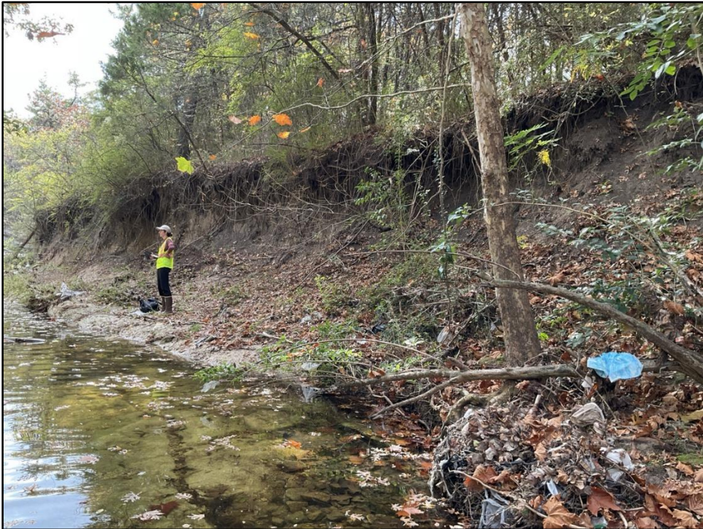
Photo 39 – STA 45+00 – Looking downstream. The right bank exhibits “Very High” BEHI rating.
