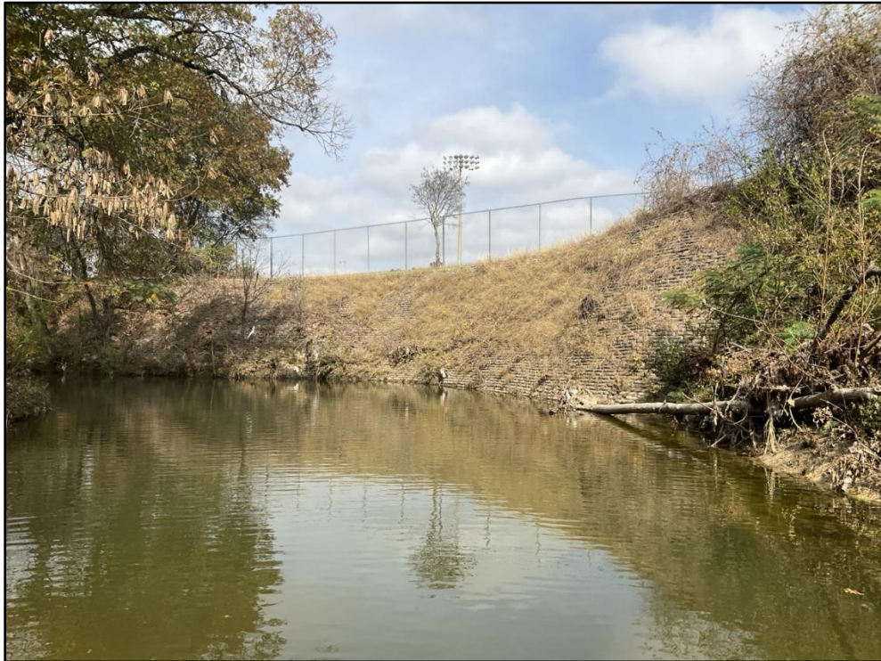
Photo 91 – STA 61+00 – Looking upstream at concrete bag wall in fair condition.
