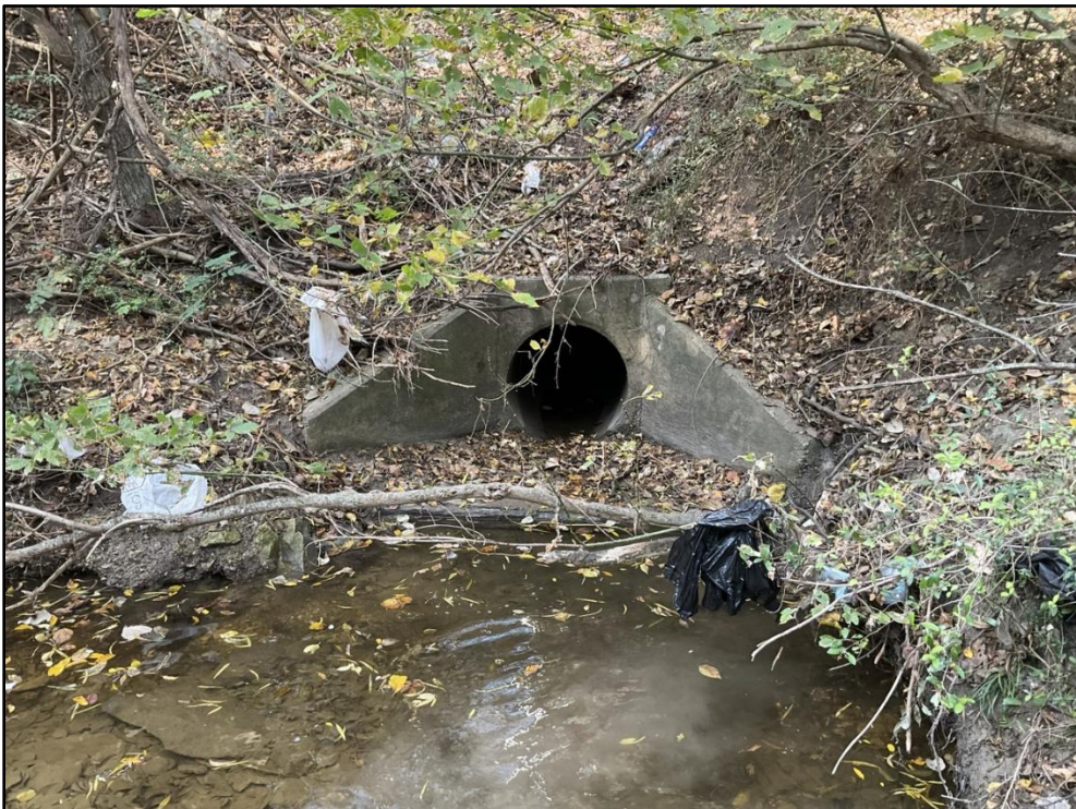
Photo 20 – STA 23+00 – 30-inch concrete stormwater outfall in good condition.
