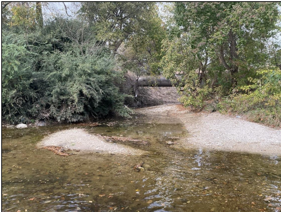
Photo 110 – STA 94+50 – Looking upstream along Mauk Branch.
