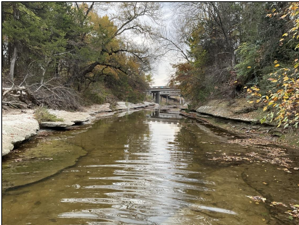
Photo 62 – STA 6+50 – Increased bedrock influence on channel bed and banks, looking downstream.
