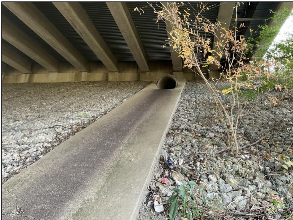
Photo 94 – STA 66+50 – 30-inch concrete stormwater outfall with flume on the right bank.
