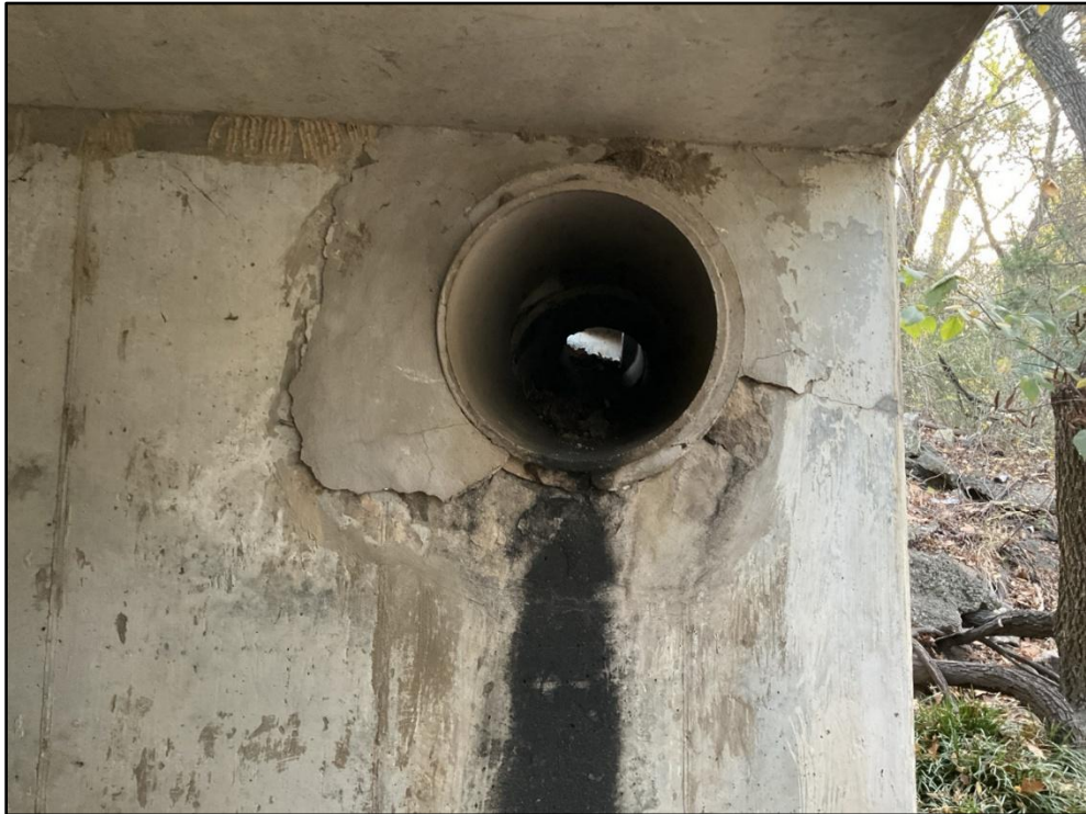
Photo 1 – STA 1+00 – 21-inch stormwater outfall inside East Wheatland Road culvert
