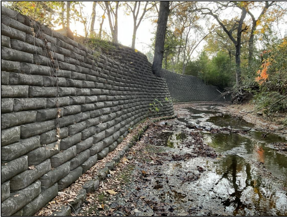
Photo 5 – Near STA 3+00 – Looking downstream along the left bank at a concrete bag wall.
