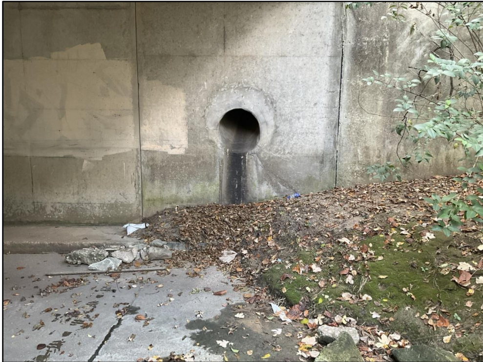
Photo 53 – STA 67+00 – 21-inch concrete stormwater outfall in right cell of East Daniieldale Road culvert.
