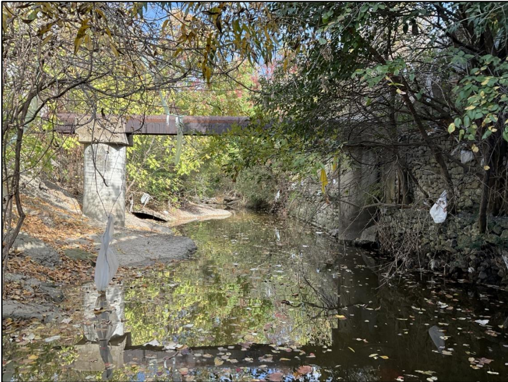
Photo 33 – STA 37+00 – Looking upstream at an 8-inch sanitary sewer crossing in fair condition. There is some local scour around the pier on the left bank and some breakage of the gabion baskets on the right bank.
