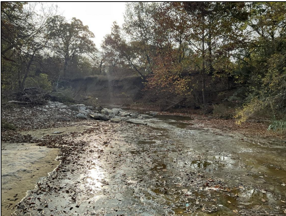
Photo 70 – STA 17+00 – Channel conditions looking downstream.
