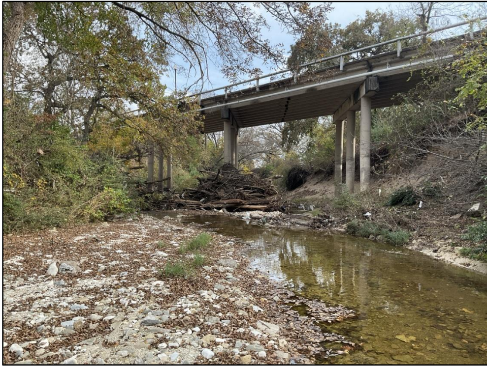
Photo 113 – STA 98+50 – Looking downstream at Wintergreen Road.
