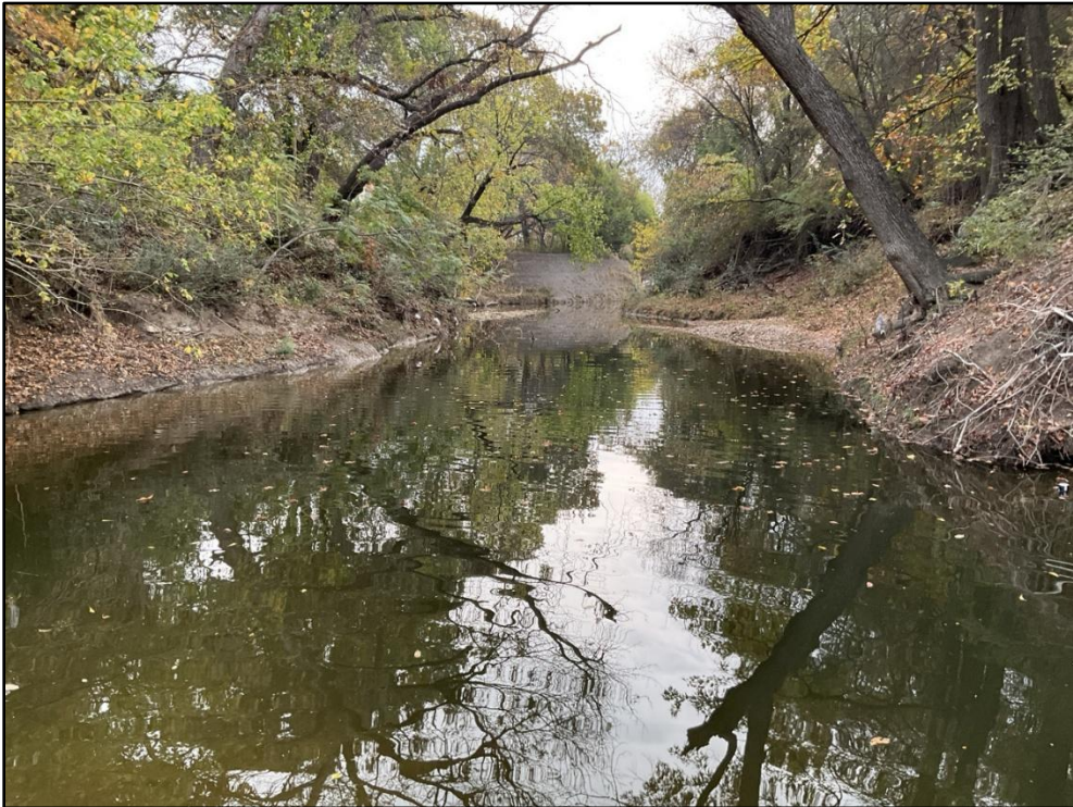
Photo 59 – Near STA 3+00 – Looking downstream at a significant scour pool.
