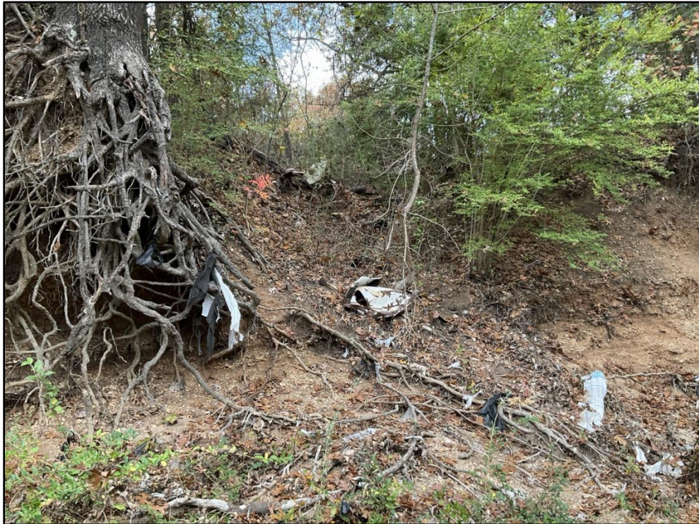
Photo 43 – STA 53+50 – Small drainage feature on right bank.
