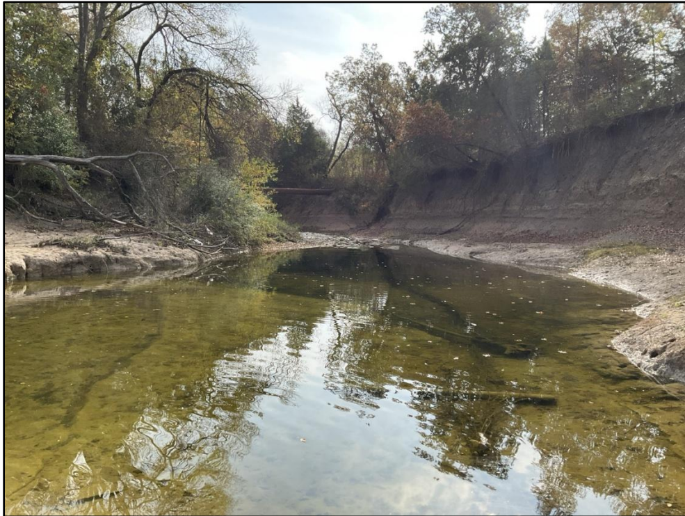
Photo 83 – STA 48+50 – Looking downstream. The right bank exhibits a “Very High” BEHI score.
