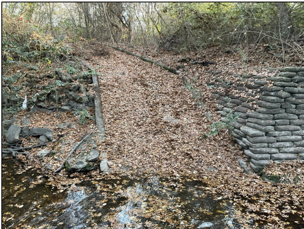
Photo 10 – STA 8+50 – Concrete stormwater flume on the left bank. 30-inch corrugated metal outfall located at the top of the concrete flume.
