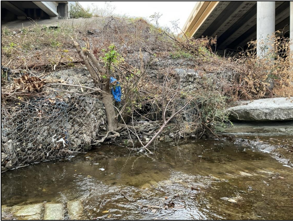
Photo 67 – STA 11+00 – 36-inch concrete stormwater outfall between gabion baskets.
