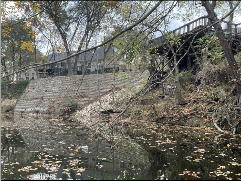
Photo 105 – STA 85+50 – Looking downstream at concrete bag wall in good condition.
