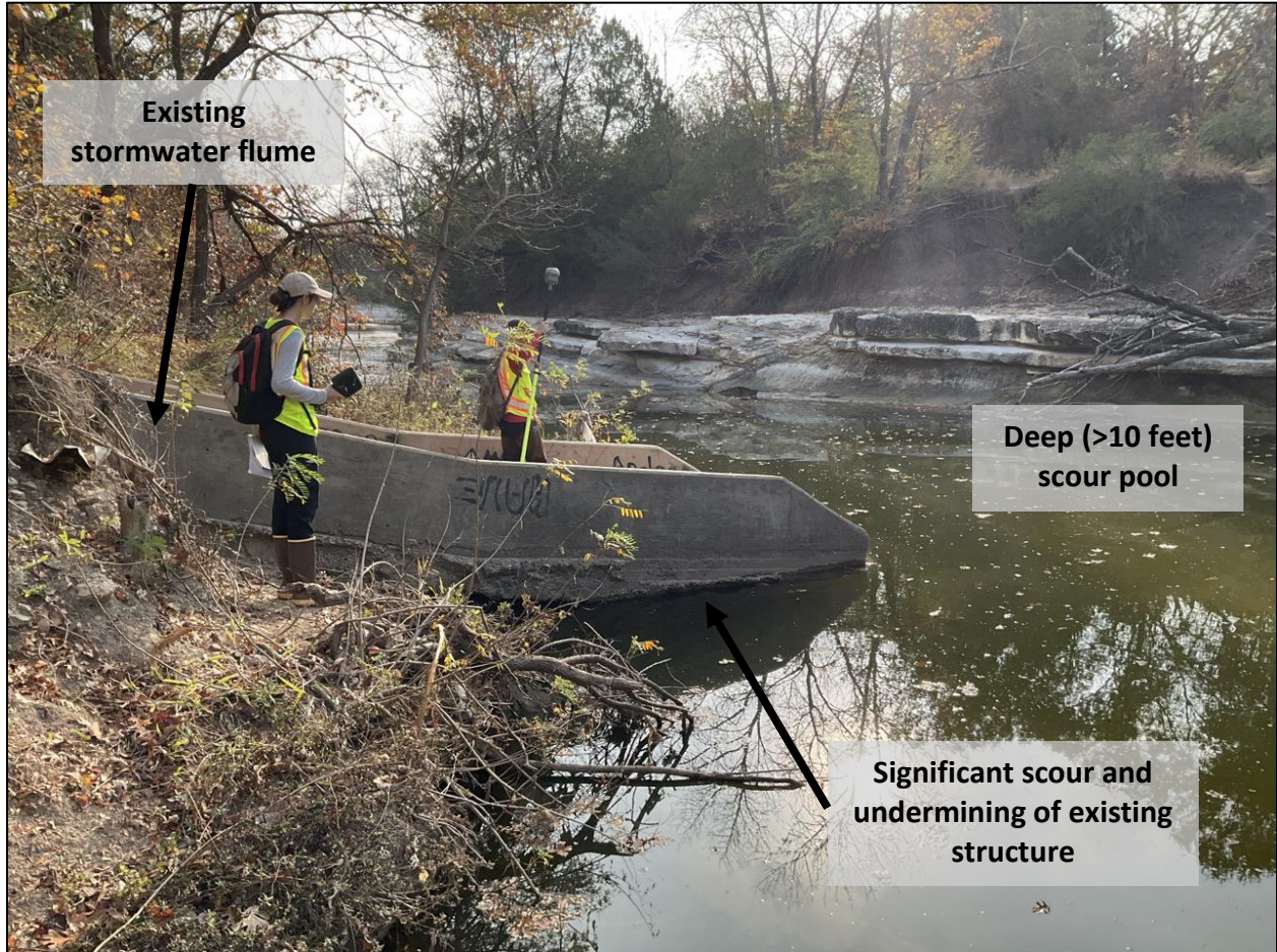
Figure 7.3 – Annotated Photograph of Area 3 Looking along the left bank of Tenmile Creek near station 28+50
