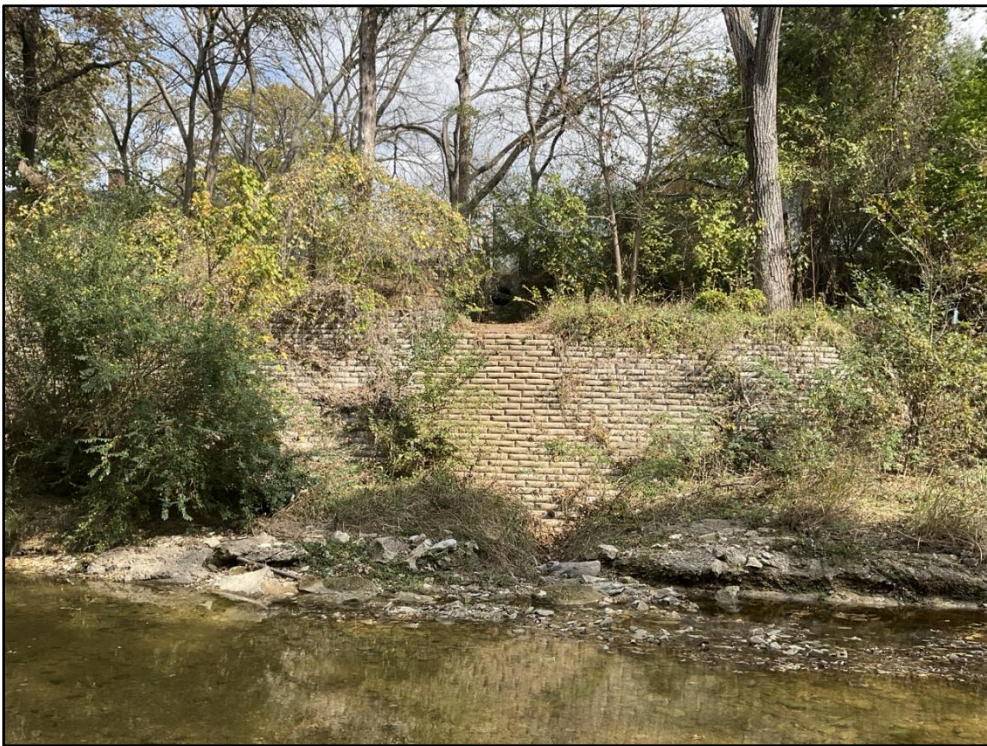
Photo 100 – STA 75+00 – 21-inch concrete stormwater outfall with flume at top of concrete bag wall.
