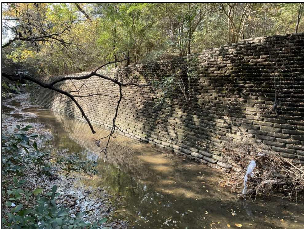
Photo 26 – STA 29+50 – Concrete bag wall in good condition.
