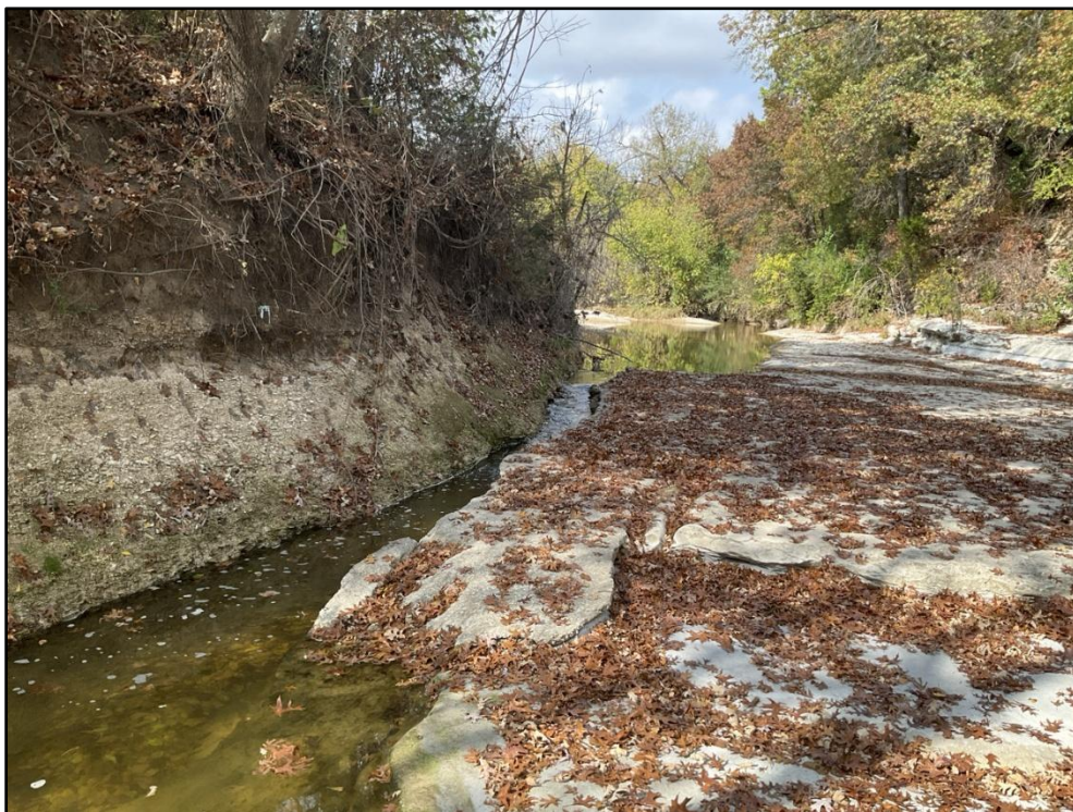
Photo 98 – STA 72+00 – Looking upstream, flow hugs right bank. A linear pour of concrete is located on the bedrock adjacent to flow.
