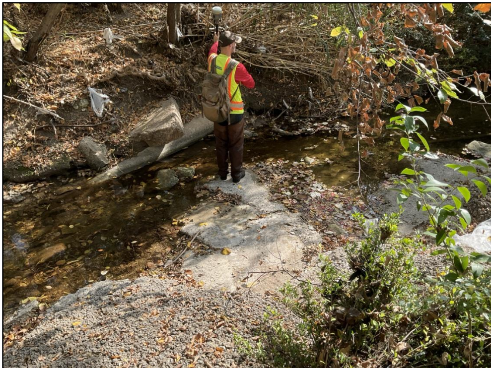
Photo 32 – STA 36+00 – Concrete encasement observed in stream bed. Some local scour of concrete, but generally in fair condition. No exposure where encasement intersects stream banks.
