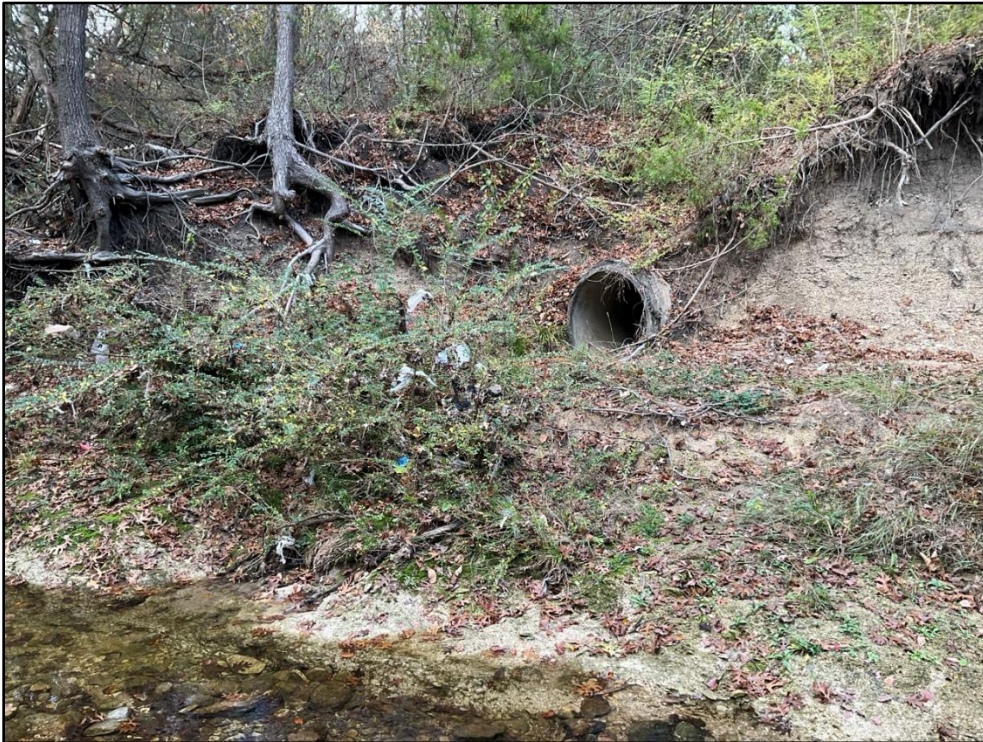
Photo 41 – Near STA 51+50 – 42-inch concrete stormwater outfall.
