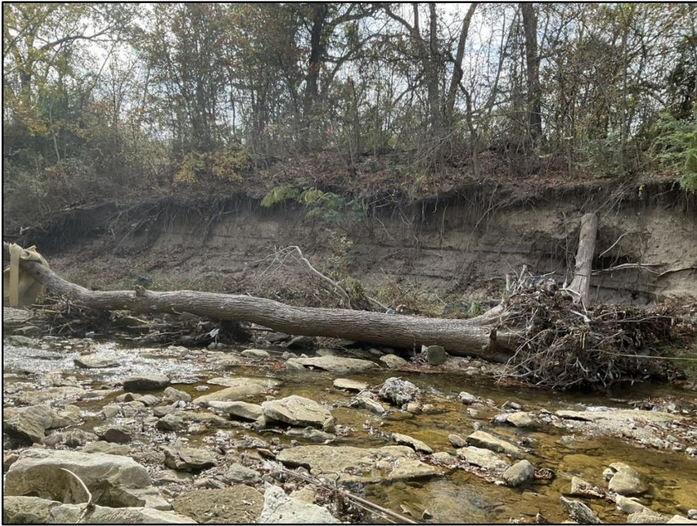
Photo 99 – STA 73+00 – Fallen tree in channel and “Very High” BEHI score.
