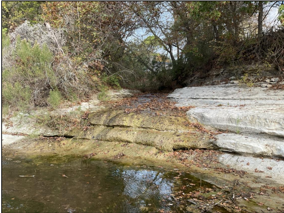
Photo 73 – STA 23+00 – Looking upstream along Tenmile Creek Unnamed Tributary 4.
