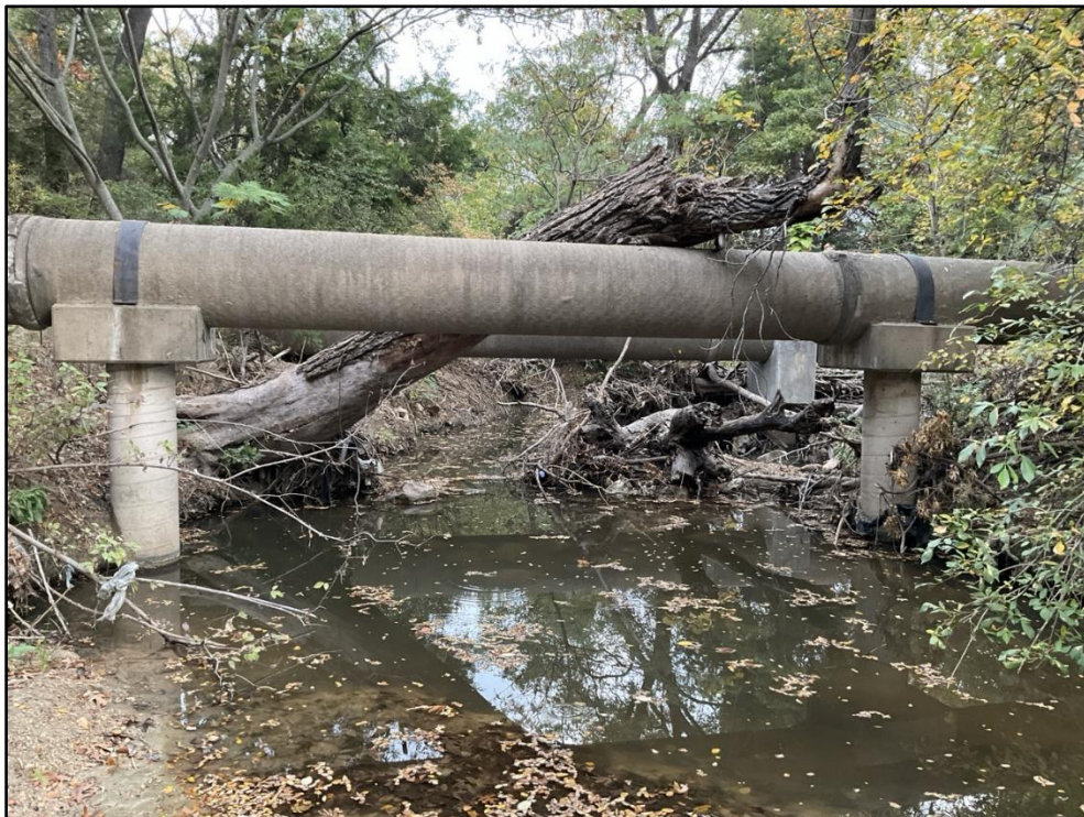
Photo 66 – Near STA 10+00 – Two 36-inch aerial sanitary sewer crossings at Horne Branch.
