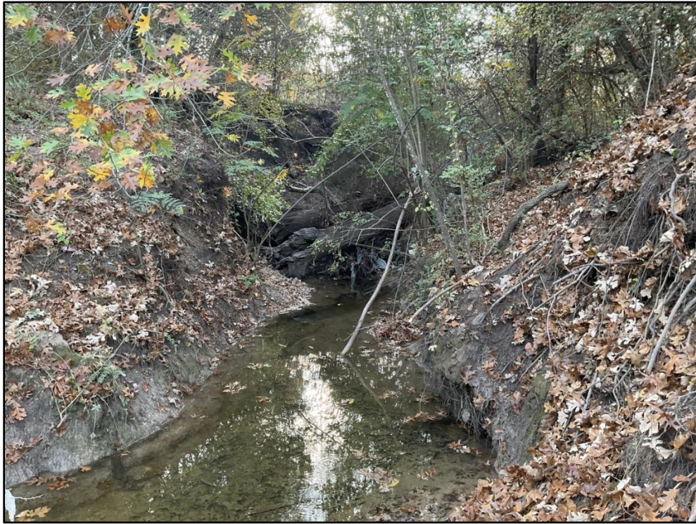
Photo 71 – STA 19+50 – Looking upstream along Tenmile Creek Unnamed Tributary 3.
